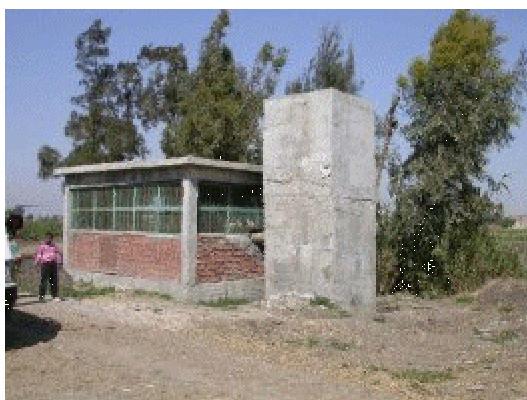
Figure 12 : Station collective de pompage Photos : S.Lanaux
